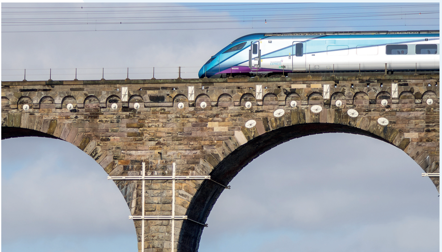
Berwick-upon-Tweed, Royal Border Bridge strengthened with 39mm Grip Bar.
