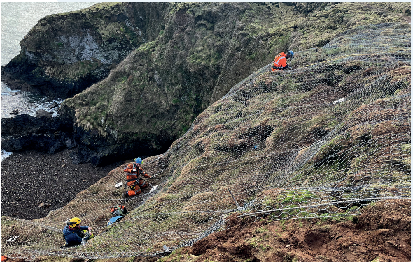
Skomer Island rock face stabilisation.
